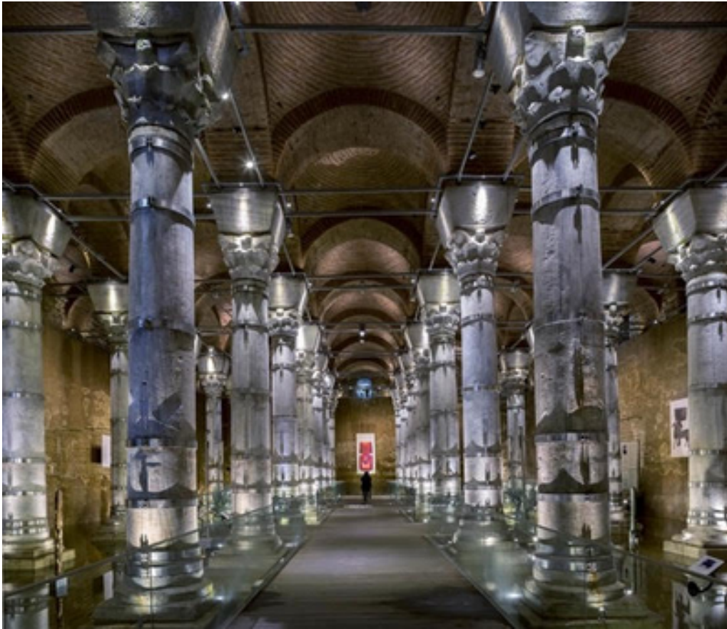
Theodosius cistern in Istanbul with steel reinforcing rings
